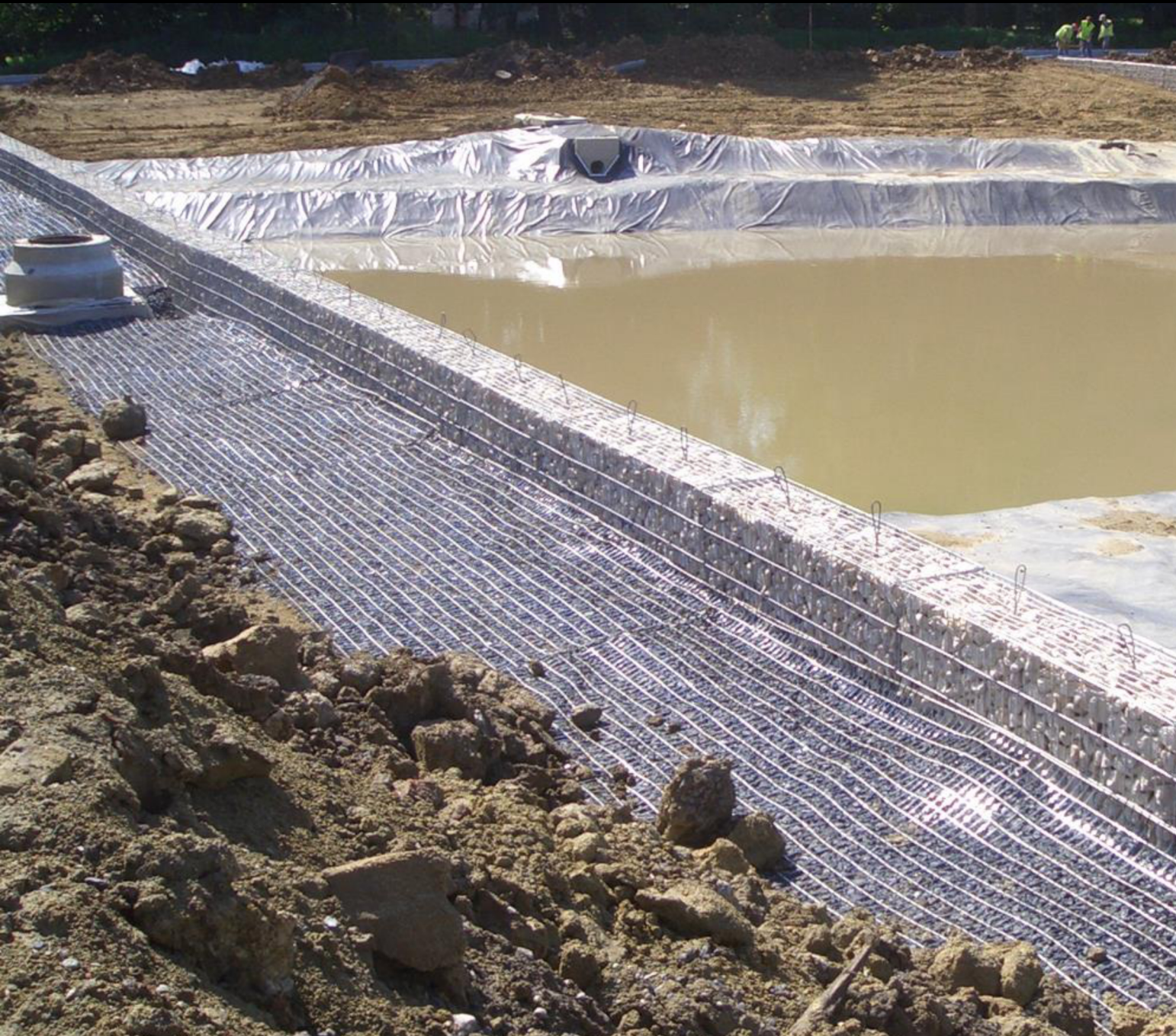
Lot 7 mur gabions
