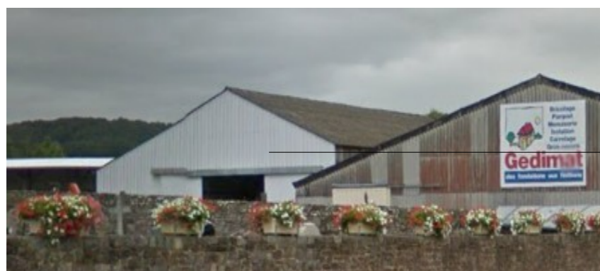
Bâtiments services techniques de Gavray
