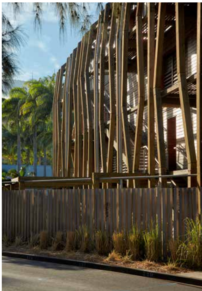
Structure apparente formant brise soleil
