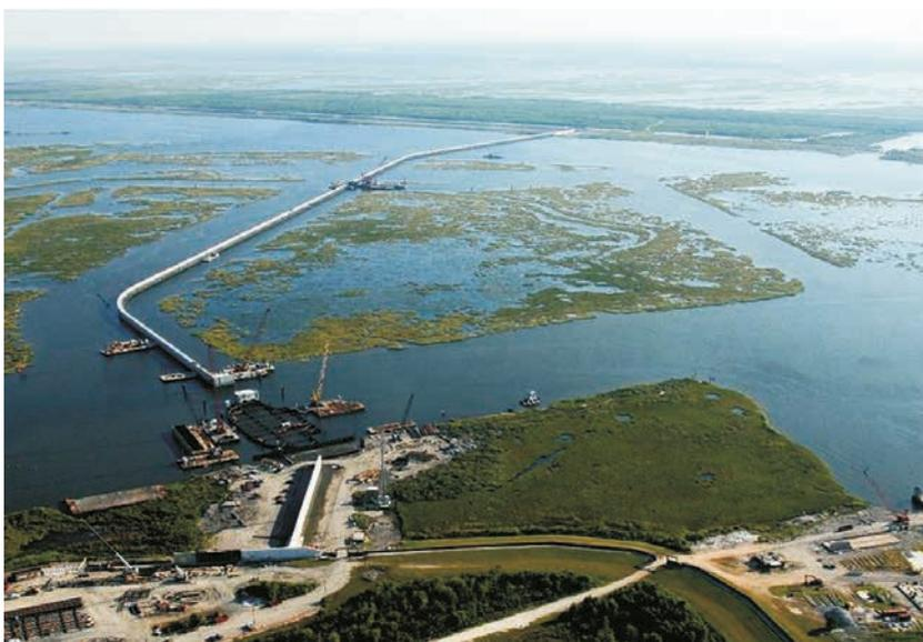
Figure 3.123 **Barrière antisubmersions**
