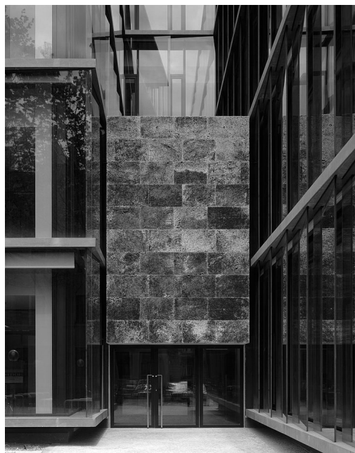
Fig.54. Munich Re Office Building, 1997-2002
