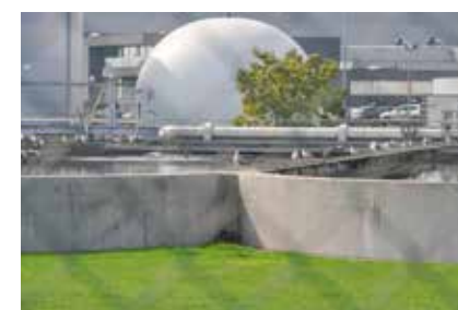
Purification artificielle Mouscron Riolwaterzuiveringsinstallatie Mouscron
