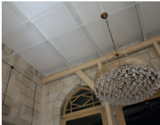
Zoom on the steel beams and the flat roof.
