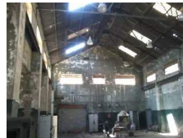
Old electricity building
