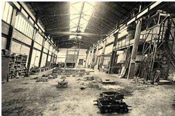
A warehouse before its renovation
