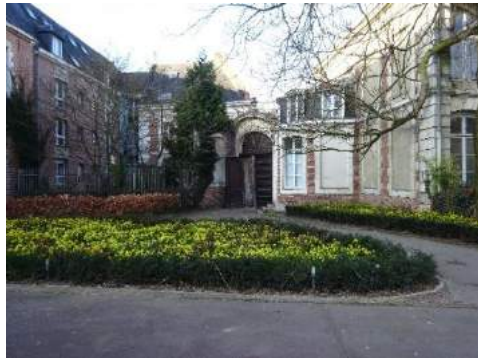
The heart of the accommodation block is opened to the public during the day, but the access is discreet (just by two doors).
