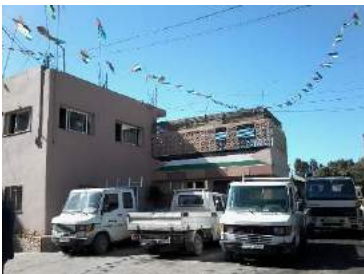
Administration building and bulldozers maintenance
