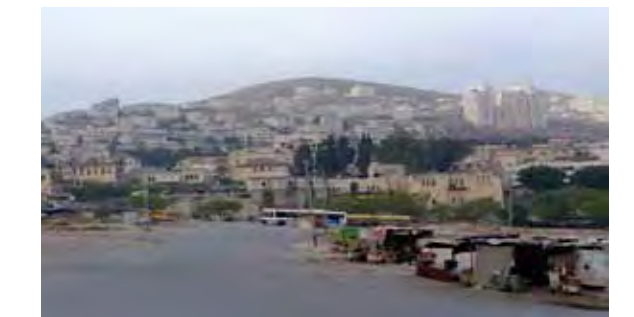
Photo 3.3 Urban Fabric in the western part of the Old City and the difference between new and old residential buildings Source: Dr. Ali Abdelrahman, 2009
