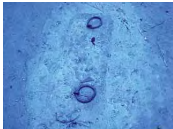
Photo 9.3 Drains covered with concrete.
