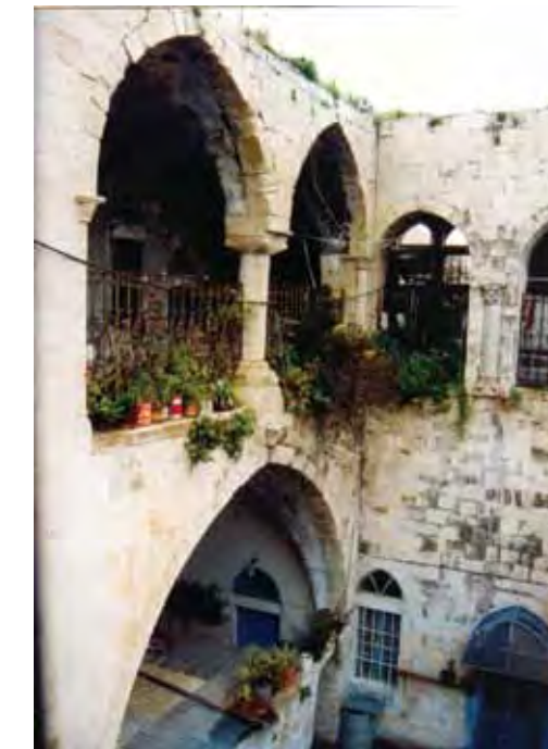
Photo 5.5 Ghazawi House. The long arched chamber ( iwan ) appears on the first floor with porticos overlooking the yard.
