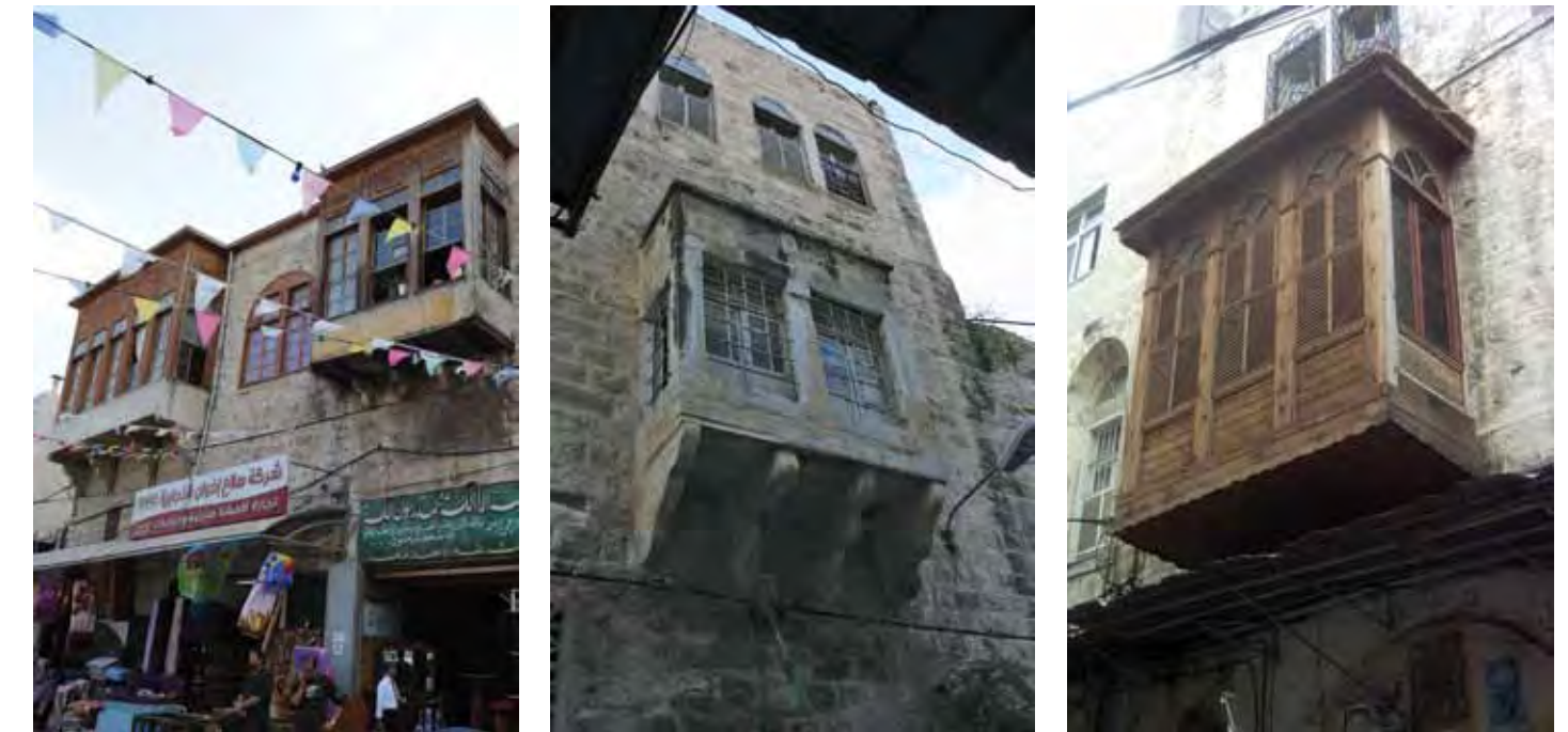
Photo 5.24 Oriel windows (Mashrabiyyat) of the houses of the Old City built of stone or wood
