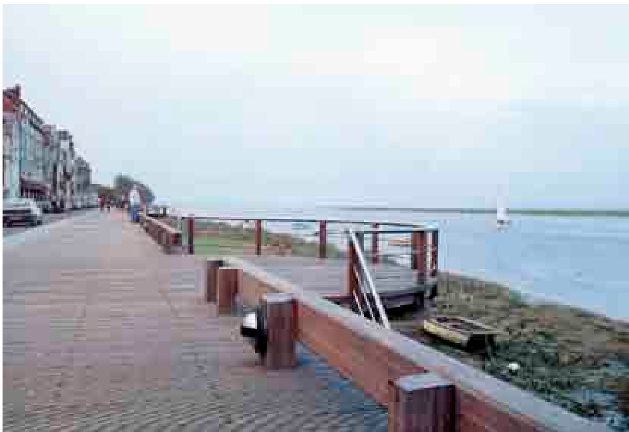
Estacade de Saint-Valery-sur-Somme. © SumProject.
